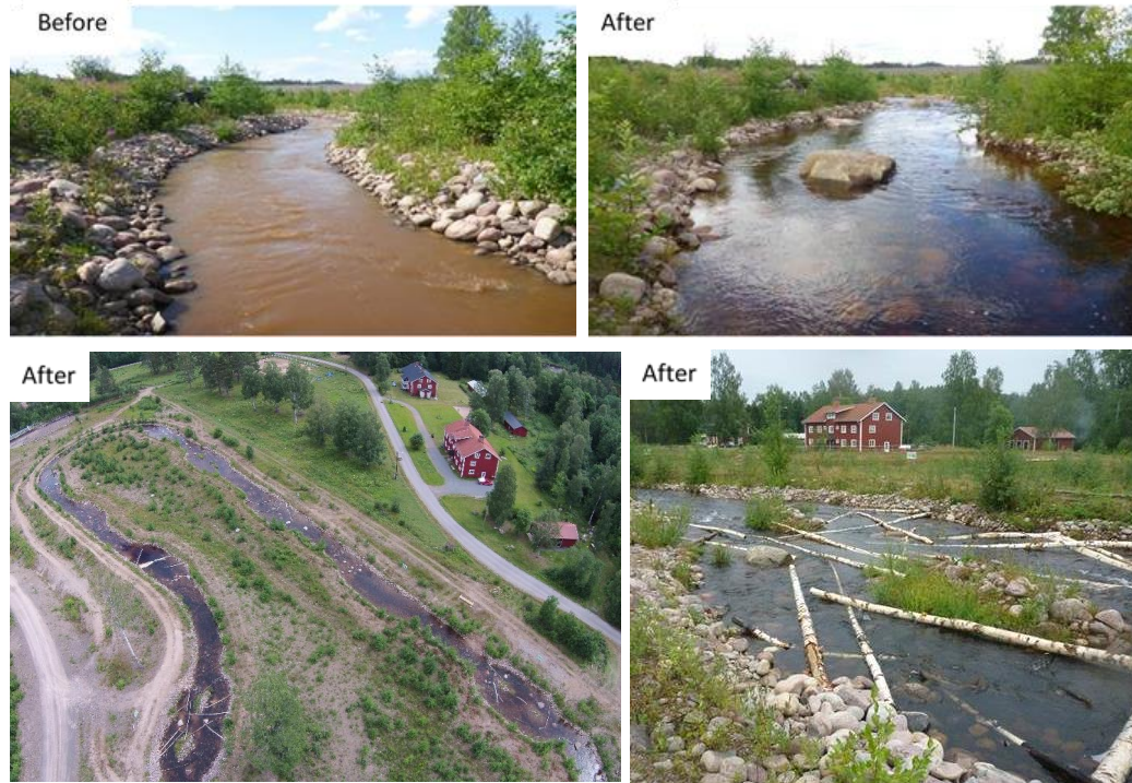
Figure 4. Modifications of the biocanal, including widening of the channel and addition of boulders, fine grain material and LWD. Photo: Anders Bruks and Stina Gustafsson
